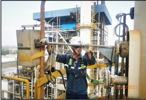
Recovery Boiler Stack
