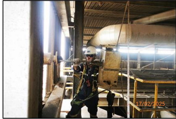
Power Boiler Stack
